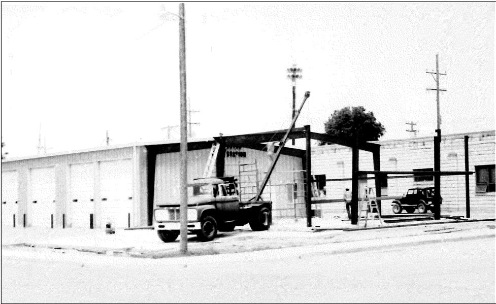
THE STEEL SUPPORT for the addition to the ambulance and fire truck barn had arrived and were put in place in the summer of 1989. This addition was to house the new fire truck and leave room to hold EMT and fire department classes.
