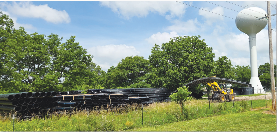
Contractors unload water line and place it near the new water tower on Ullery Road constructed for Linn Valley. Water lines will be connected to transmission lines behind Stainbrook’s in La Cygne to bring La Cygne water to the water tower.
